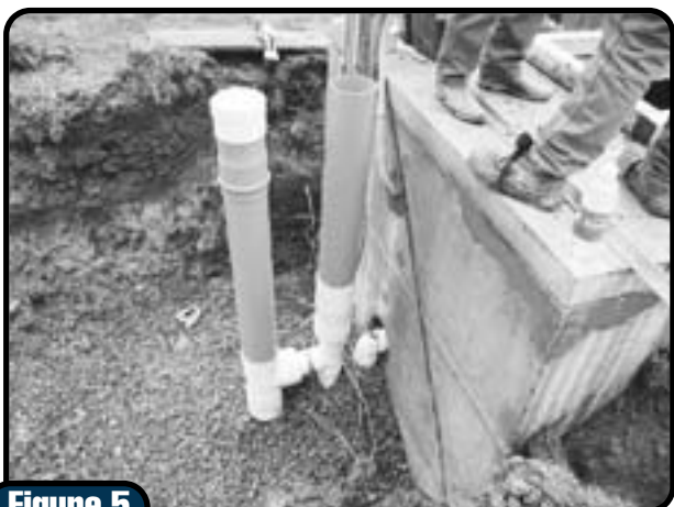
Figure 5 Side view of a residential UV unit Photo courtesy of Ashco – A Corp., Morgantown, WV
