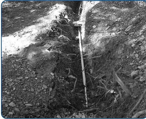
This photo shows a water line crossing under a sewer line. This arrangement violates health codes in every state because a sewer leak could contaminate the water line below. (Photo by Allen Marchan)
