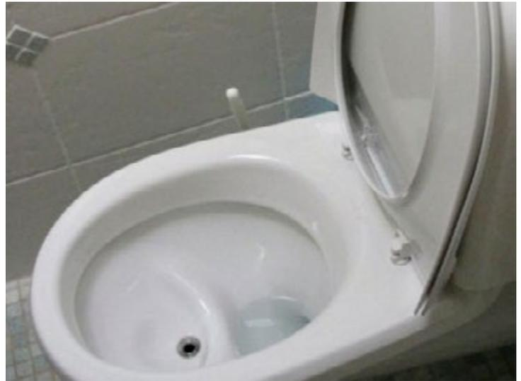
*Urine-diverting toilets have a vertical barrier in the bowl that separates urine (front section) from other toilet waste. Low-flow and waterless urinals can also be used to divert and collect urine from men's restrooms.*
