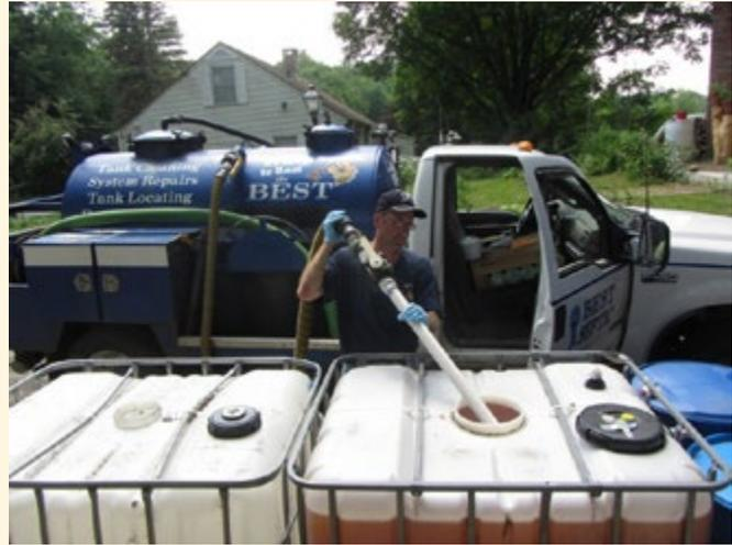
*As part of the Rich Earth Institute project, Seth True, of Best Septic, pumps from a 275 gallon collection tank. A family of three can fill a tank this size in eight months.*
