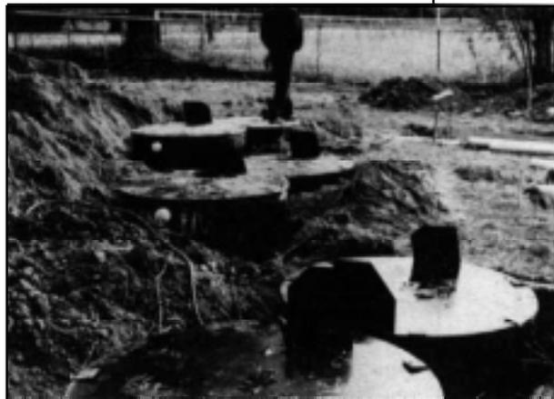
◀ **PHOTO 2** Installing septic tanks (January, 1995).
