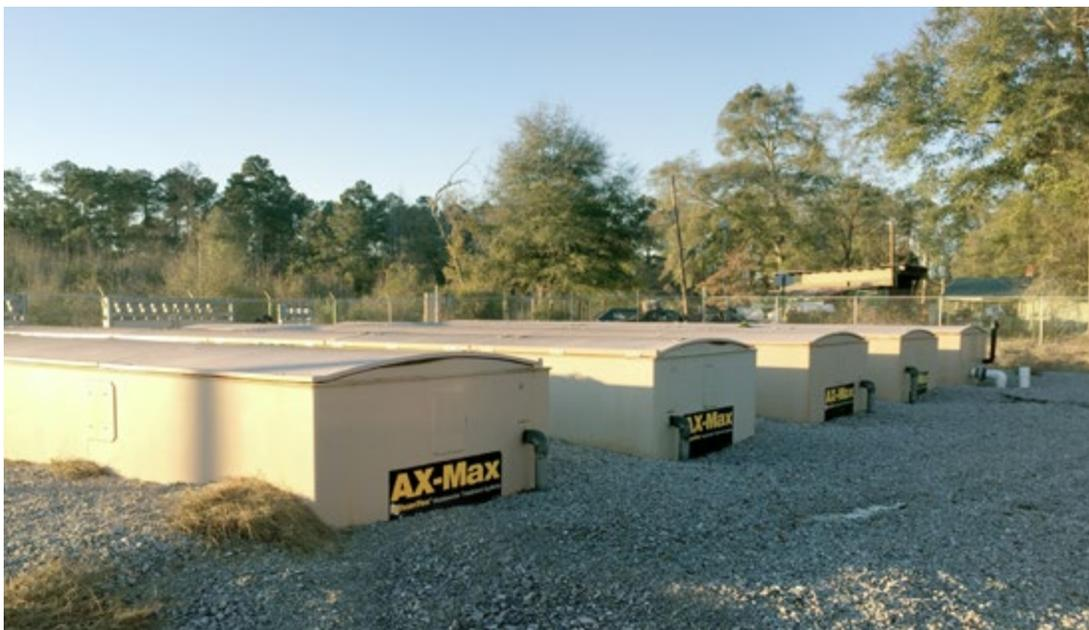
*Although Fulton's five AX-MAX™ units are situated partially above-ground, they can also be installed in-ground, as well as individually or in multi-tank arrays.*
