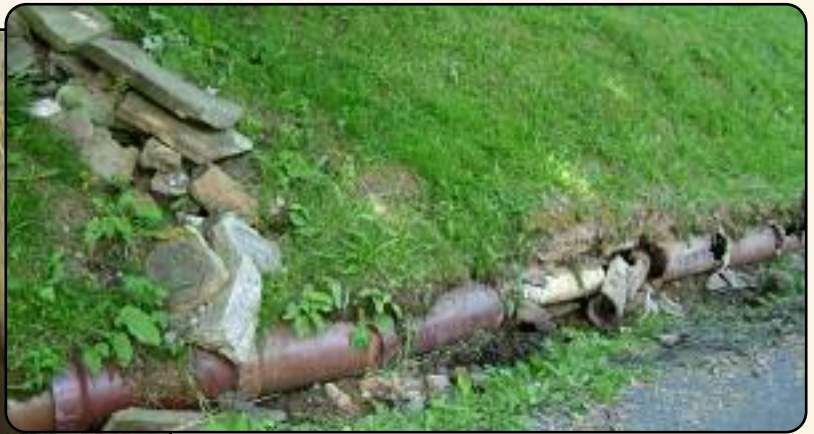
The photo above shows decaying 20th-century water supply pipe. To the left, a water sump for a 19th-century wind-powered system is shown.
