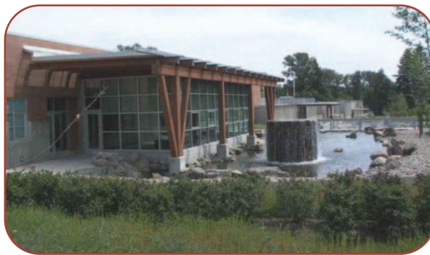
Photos Source: Wilsonville, Oregon Water Treatment Plant
