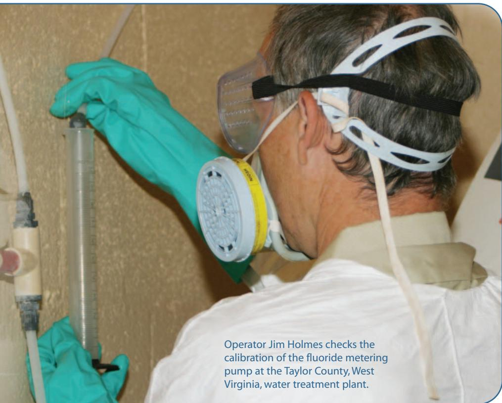
Operator Jim Holmes checks the calibration of the fluoride metering pump at the Taylor County, West Virginia, water treatment plant.
